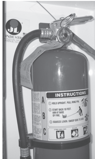
Figure 4.22 Type A-B-C fire extinguisher
